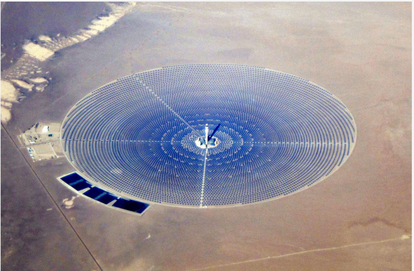
Crescent Dunes Solar Energy Installation , situated in Nevada, uses its CSP array to heat molten salt flowing in the tower at the center of the array. Heat energy is stored in the molten salt and can be used to power steam generators.
