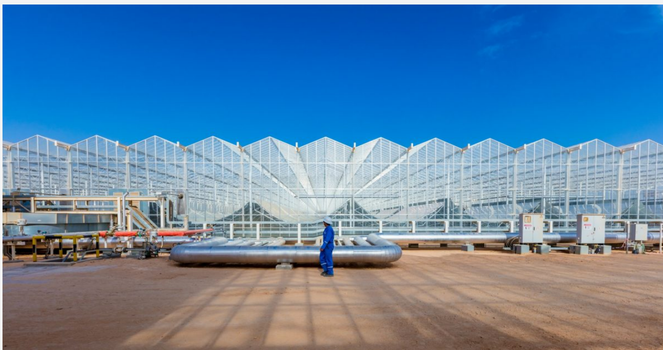
GlassPoint Solar's Miraah plant in Oman went operational in 2017. Source: GlassPoint Solar
