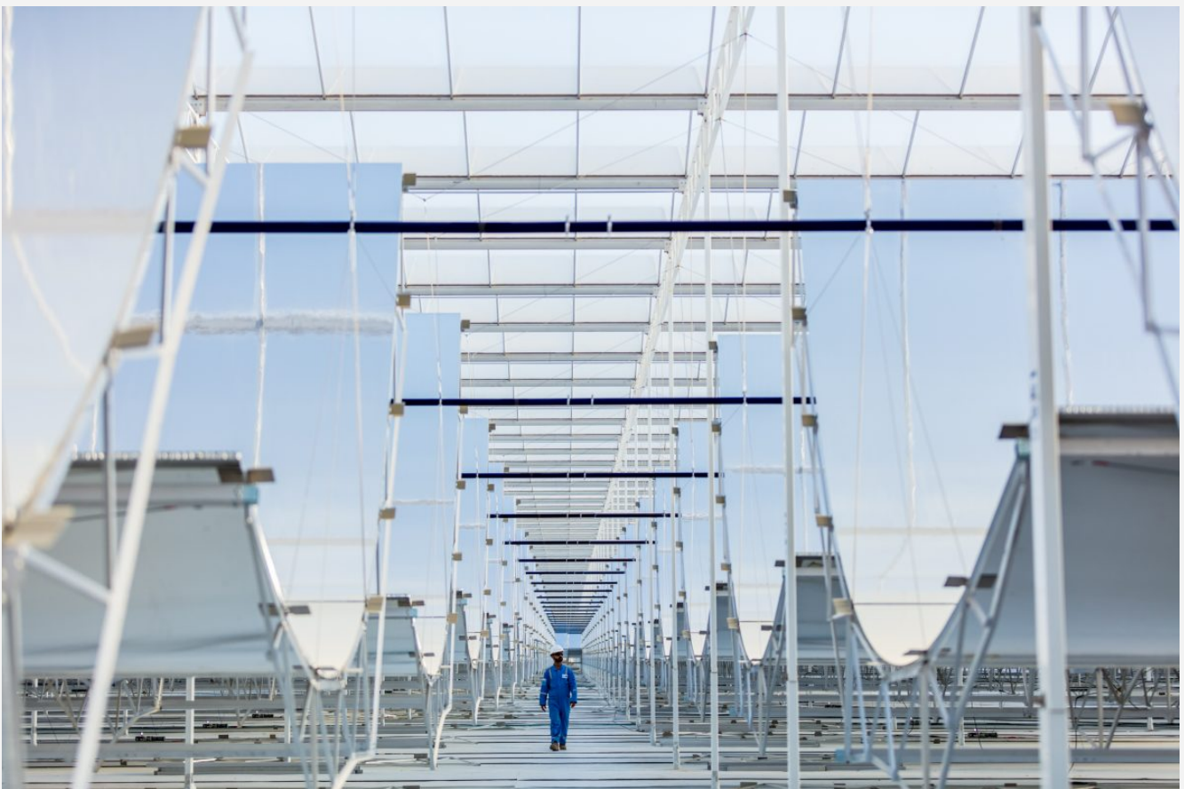
A worker walking through the Miraah facility. Note the trough-shaped reflectors and the roof of the greenhouse. Source:
